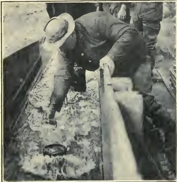
CLEANING-UP THE SLUICES.
